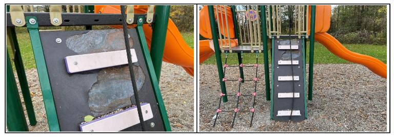
**Rappel wall -** The plastisol coatings on the rappel wall were peeling at the time of inspection. Monitor the conidtion and repair as required.
