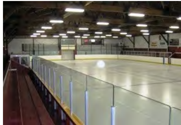
Existing Ice Pad at NDCC
