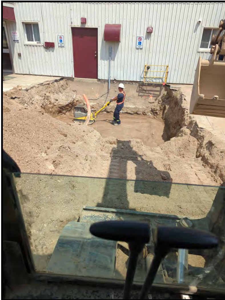
Figure 4: Compacting Backfill Material. Facing East.
