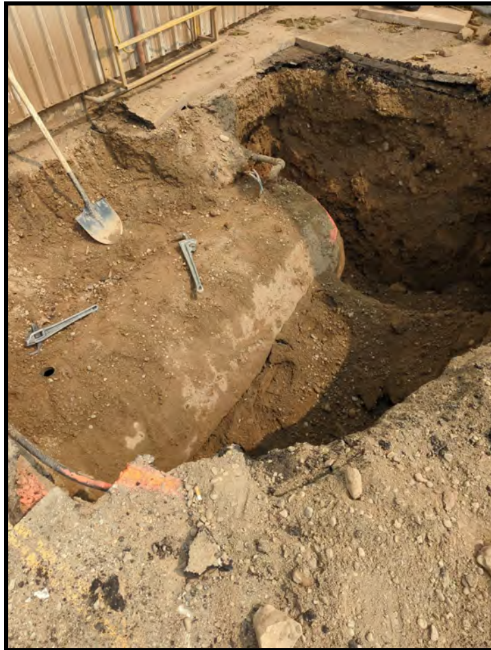
Figure 3: Underground Storage Tank Location. Facing Southeast.
