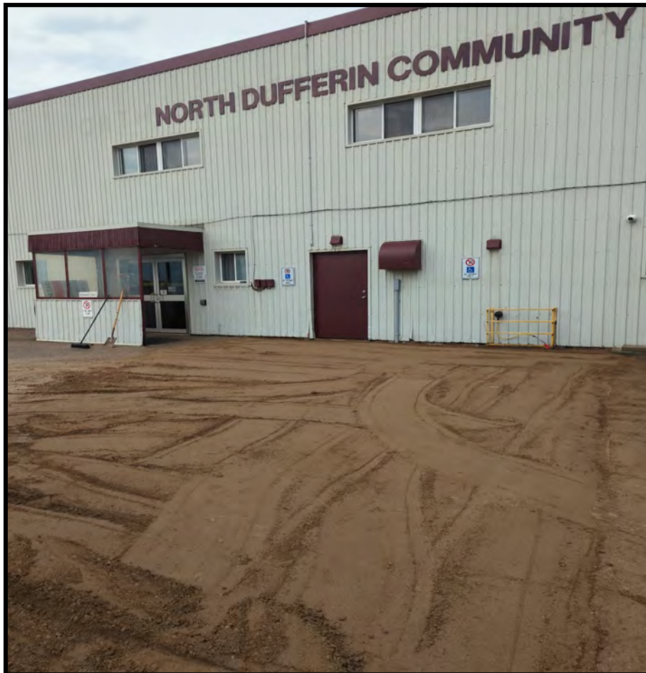
Figure 5: Backfilled Area. Facing Northeast.
