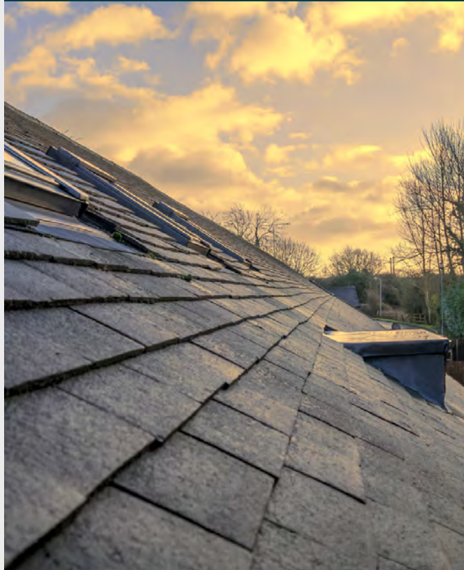
Admin Building Roof Replacement
