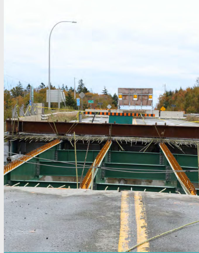
Bridge & Culvert Rehabilitation
