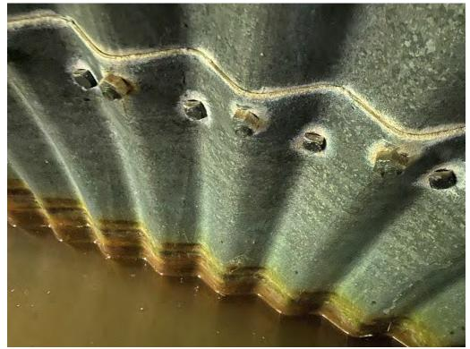
Barrels - Incorrect Bolting Pattern, Rust Staining at Waterline
