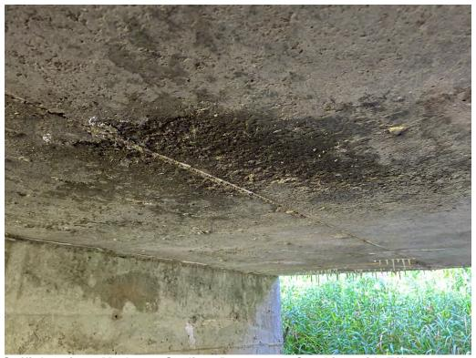
Soffit Interior - Moderate Scaling, Dampness, Cracking with Efflorescence
