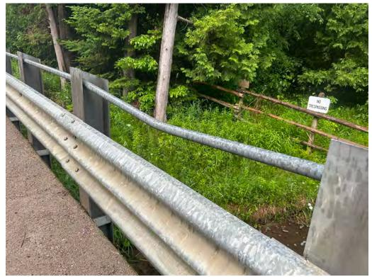
Deck Guide Rail - Minor Impact Damage
