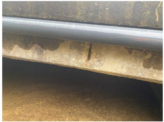
Soffit Exterior – Spall With Exposed Corroded Rebar
