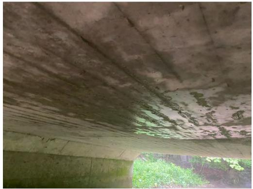
Soffit (Interior) - Medium Cracks, Dampness
