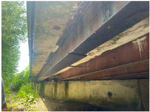
Girders Middle - Severe Rusting & Corrosion
