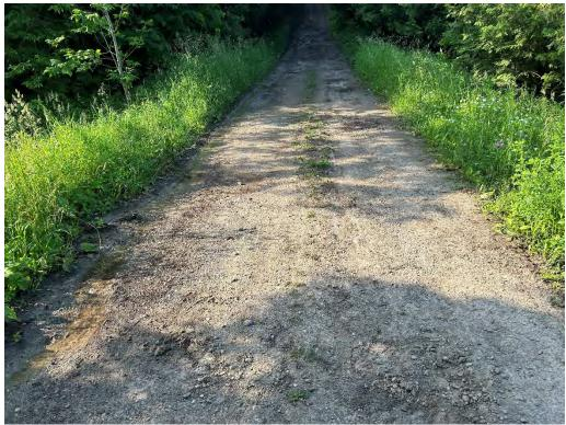
Deck Wearing Surface – Washouts Between Culverts on Shoulder, Loose Gravel, Light Wheel Track Rutting
