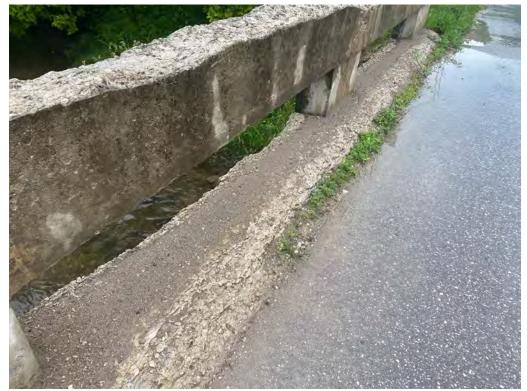
Barrier Wall - Disintegration, Spalling and Scaling
