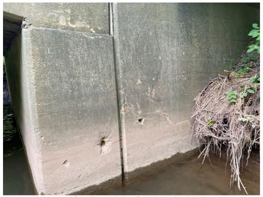
Wingwalls - Spalling, Hairline Cracking with Efflorescence
