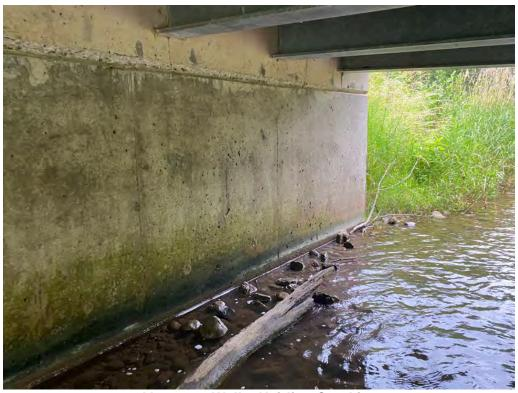
Abutment Wall - Hairline Cracking
