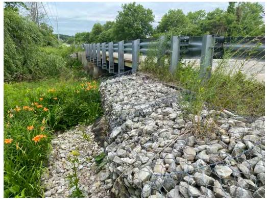
Retaining Wall - Rotation and Bulging
