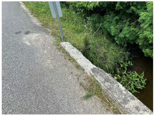
Curbs - Disintegration, Delamination
