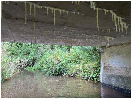
Soffit Interior - Cracking with Moisture Penetration, Stalactites
