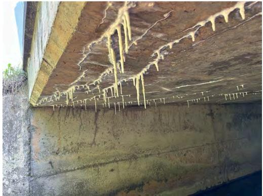
**Soffit Exterior – Moisture Penetration & Stalactites**
