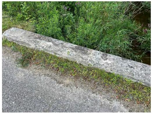
Curbs – Disintegration & Stained Cracking Throughout
