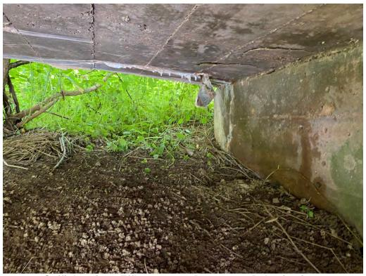
Soffit Interior – Efflorescence, Dampness, Delaminations
