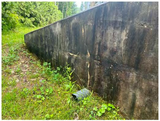
Wingwall - Hairline Stained Cracks
