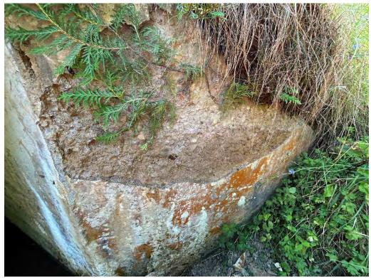
Wingwalls - Disintegration, Delamination & Spalling
