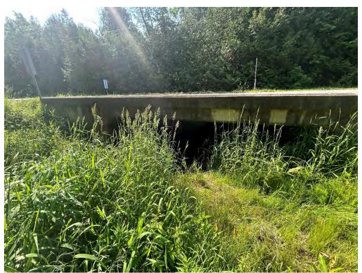
Embankments – Vegetation Growth Restricting Inlet Flow, Minor Washouts at Curb Corners
