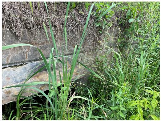
Wingwalls - Overgrown in Vegetation, Delaminations, Stained Cracking, Scaling
