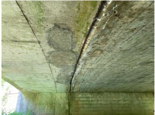
Soffit Interior - Concrete Patches, Stained Cracks with Efflorescence
