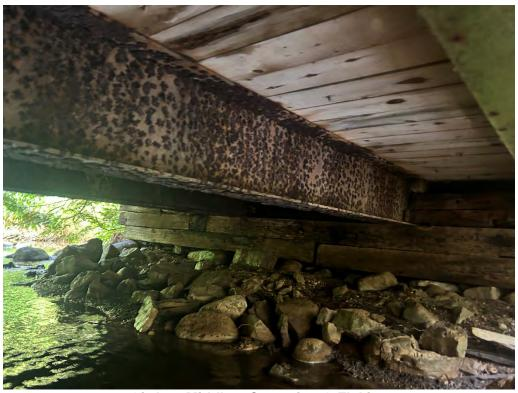
Girders Middle - Corrosion & Flaking
