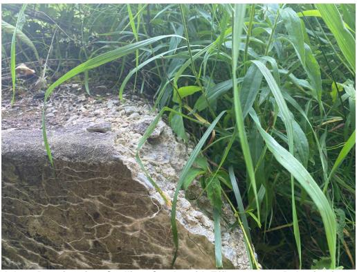
Inlet - Deterioration, Spalling, Cracks with Efflorescence, Delaminations
