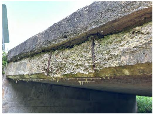
Soffit Exterior – Severe Disintegration with Exposed Corroded Rebar, Efflorescence
