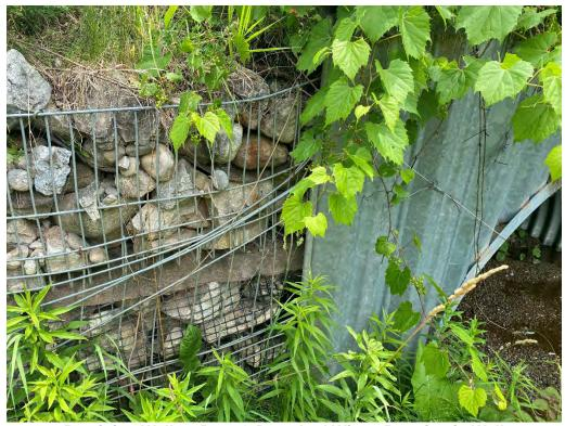
Retaining Walls - Bent & Detached Wires, Rotation in Wall
