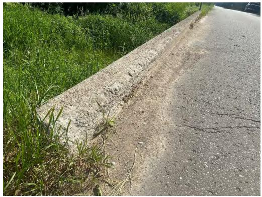
Curbs – Spalling & Disintegration, Narrow Cracking
