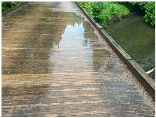
Deck Top - Moderate Rotting, Water Ponding
