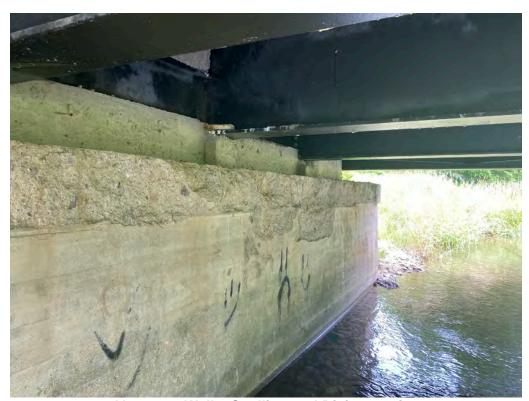
Abutment Wall – Spalling and Disintegration
