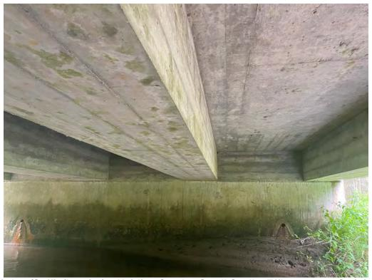
Girders/Soffit (Interior) - Hairline Cracks, Small Spalls, Efflorescence Staining
