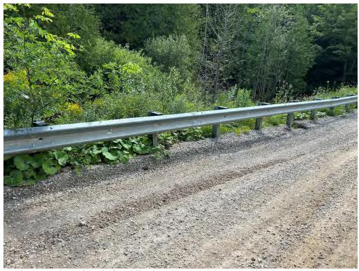
Approach Guide Rail - Missing Plough Markers, Washouts at Posts
