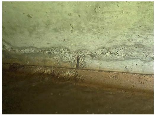
Barrel – Honeycombing, Exposed Corroded Rebar
