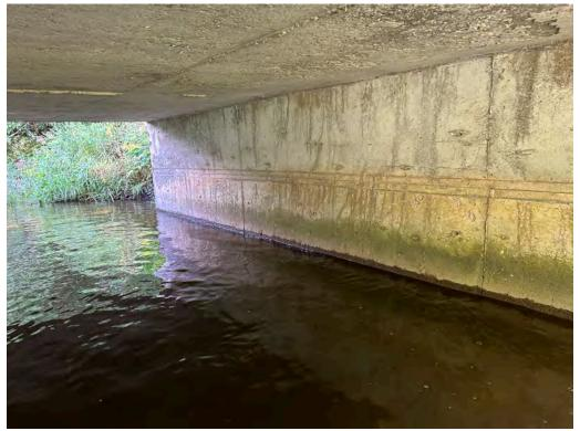
Abutments - Narrow Vertical Stained Cracks, Staining at Waterline
