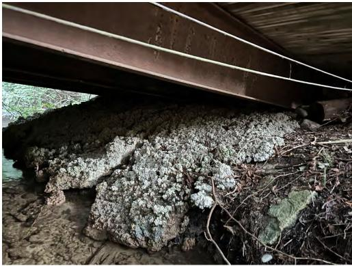
Abutments – Mass Concrete Poured on Slopes, Undermined & Wide Cracks Through Middle
