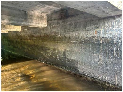
Abutments - Narrow Vertical Stained Cracks,
