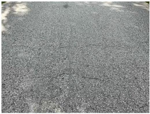
Deck Wearing Surface - Minor Settlement, Light Transverse Cracking
