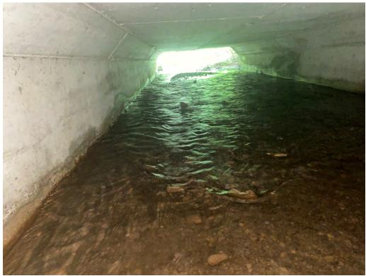
Barrel - Deterioration at Waterline
