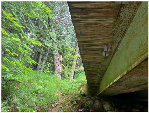
Soffit (Exterior) - Rot, Moisture Penetration
