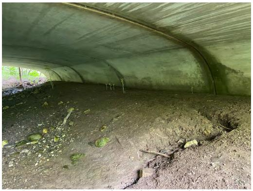
Barrel - Moisture Penetration at Joints, Aggregation Build-Up
