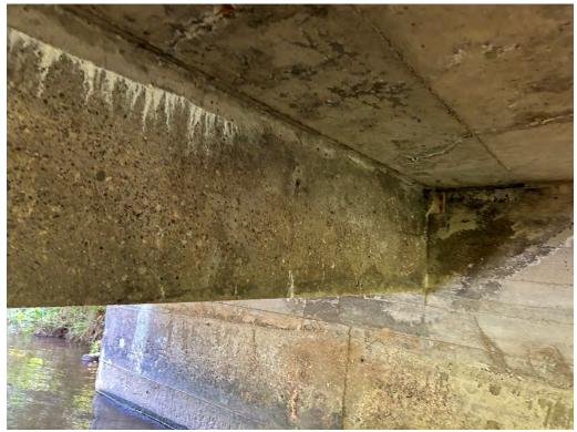
Girder Ends - Medium Cracks, Efflorescence, Spalls
