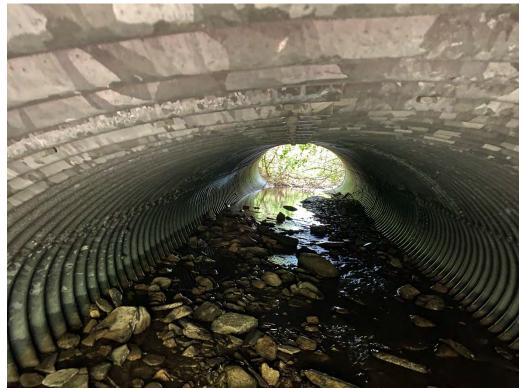
Barrels - Plate Deformations, Cusping, Corrosion at Water Line
