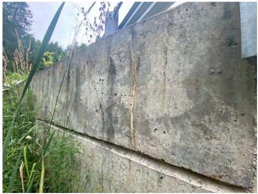
Wingwall - Vertical Cracks with Efflorescence Staining
