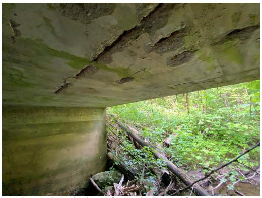
Barrel - Delaminations & Spalls with Exposed Corroded Rebar
