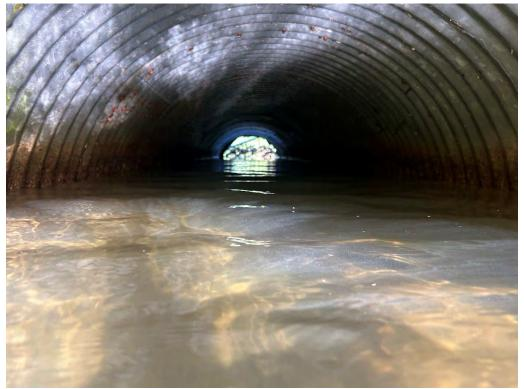
Barrels - Corrosion at Bolts & Waterline
