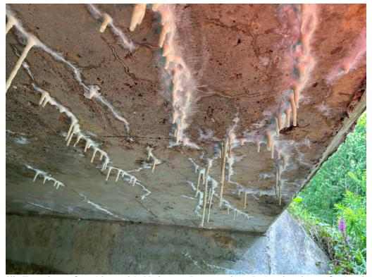
Soffit Exterior - Cracking with Moisture Penetration, Delaminations, Stalactites
