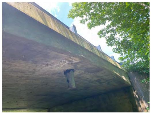
Soffit Exterior – Moisture Penetration Through Concrete Patches
