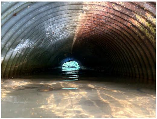
**Barrels – Moderate to Severe Corrosion Along North Section**
