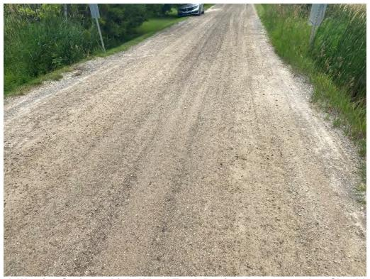
Deck Wearing Surface - Light Wheel Track Rutting, Loose Gravel on Shoulders
