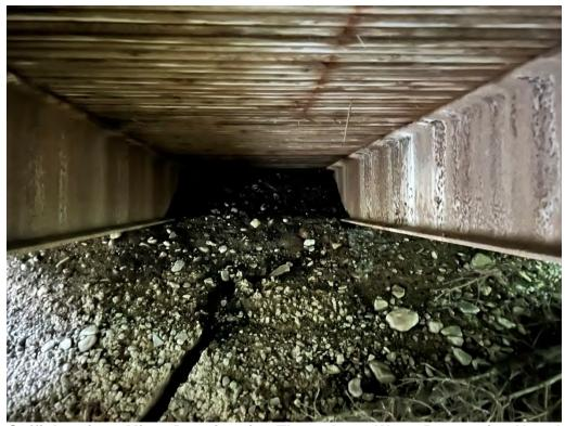
Soffit Interior - Minor Deterioration Throughout, Water Penetration Noted
