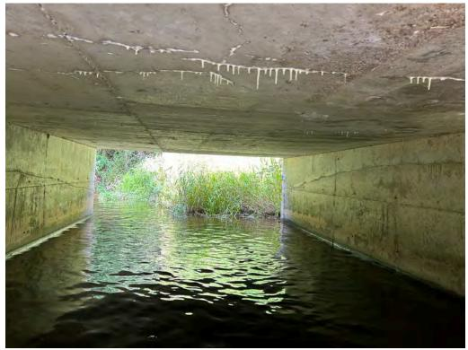
Soffit Interior - Cracking with Moisture Penetration, Stalactites, Light Scaling
