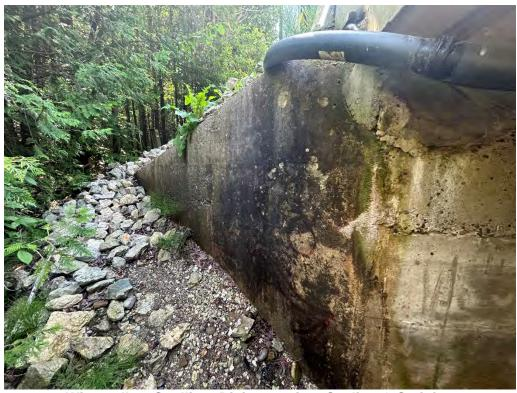
Wingwalls - Spalling, Disintegration, Scaling & Staining
