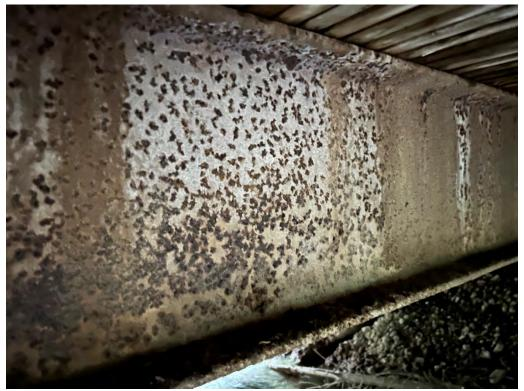
Girders Middle - Corrosion & Flaking
