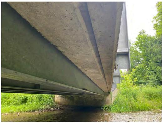
Soffit (Exterior) - Narrow Stained Cracking
