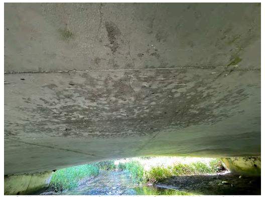
Soffit Interior - Narrow Cracking, Light Scaling & Moisture Staining
