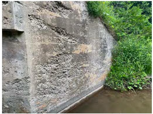
Wingwall – Severe Scaling, Disintegration
