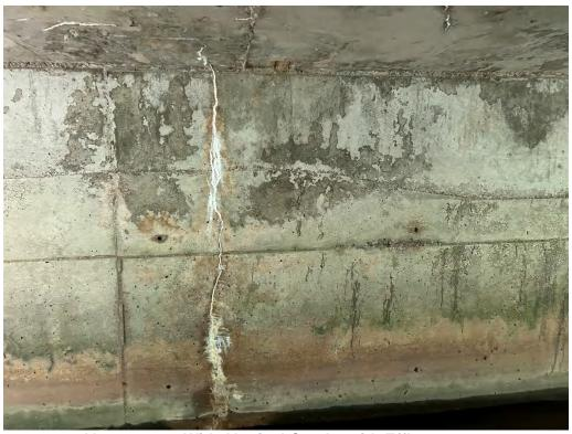
Abutments - Wide Vertical Cracks with Efflorescence
