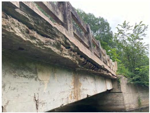
Soffit/Curb (Exterior) – Severe Disintegration of Concrete with Exposed Corroded Rebar
