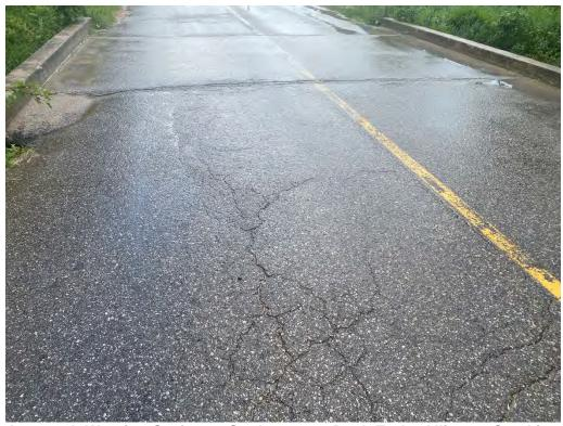
Approach Wearing Surface - Settlement at Deck Ends, Alligator Cracking
