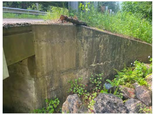
Wingwall - Hairline Stained Cracks
