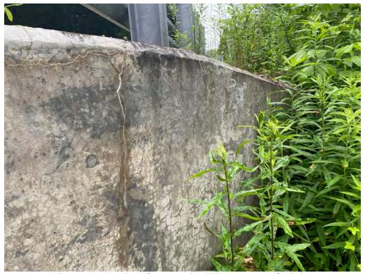
Wingwall – Vertical Cracks with Efflorescence Staining
