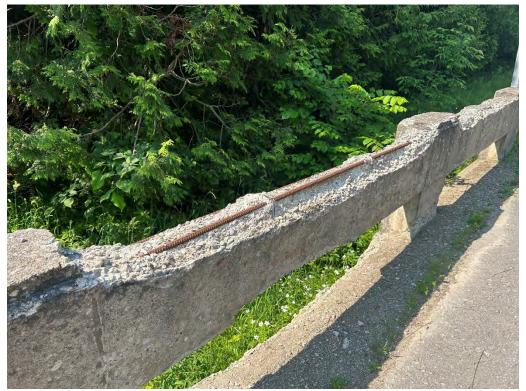
Barriers - Severe Disintegration, Exposed Corroded Rebar, Delaminations
