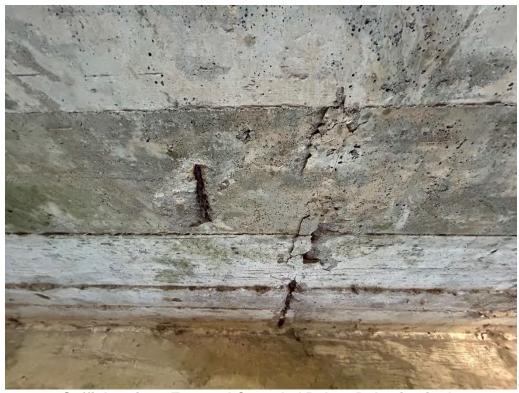
Soffit Interior - Exposed Corroded Rebar, Delamination's
