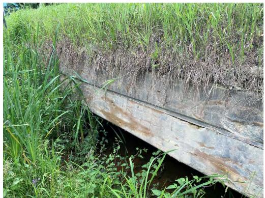
Soffit Exterior – Severe Disintegration, Delaminations, Stained Cracking Throughout
