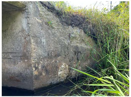
Wingwalls – Severe Disintegration with Exposed Corroded Rebar
