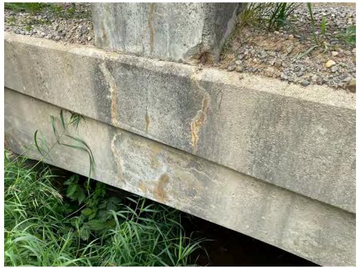
Soffit Exterior – Stained Cracking Throughout
