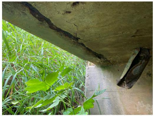
Soffit Exterior – Spalls with Exposed Corroded Rebar, Deck Drains not Functional
