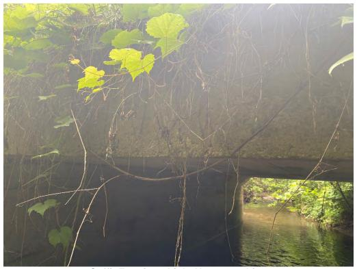
Soffit Exterior - Light Honeycombing
