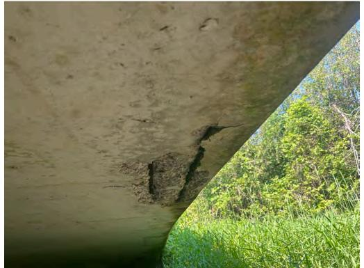
Soffit Exterior - Spalling with Exposed Corroded Rebar, Delaminations, Staining
