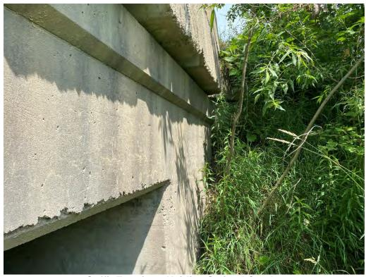
Soffit Exterior - Hairline Stained Cracks
