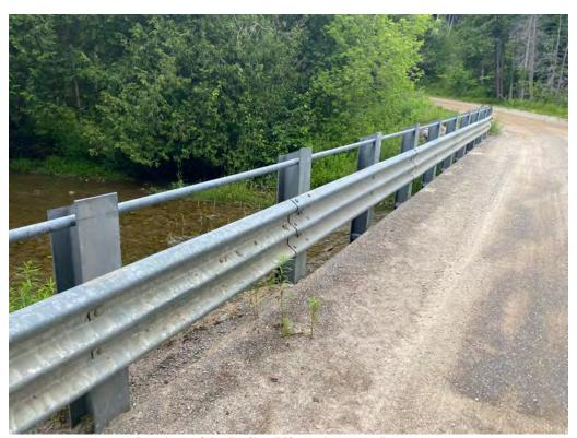
Deck Guide Rail - Minor Impact Damage
