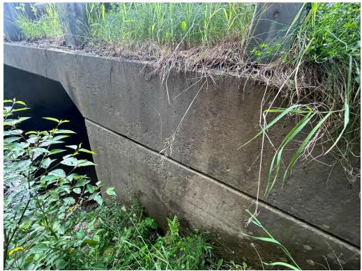
Wingwalls - Light Scaling, Hairline Cracking, Scouring
