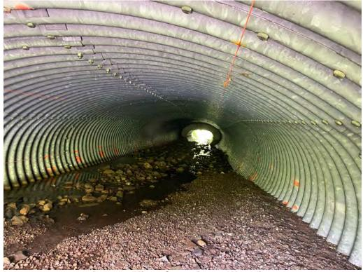
**Barrel – Minor Corrosion at Waterline**
