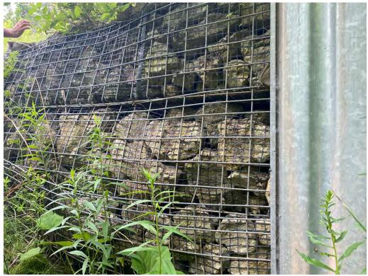
Retaining Walls - Bulging & Settlement
