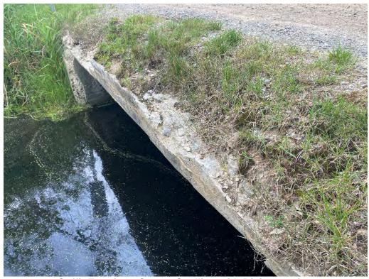
Soffit Exterior – Severe Spalling with Disintegration
