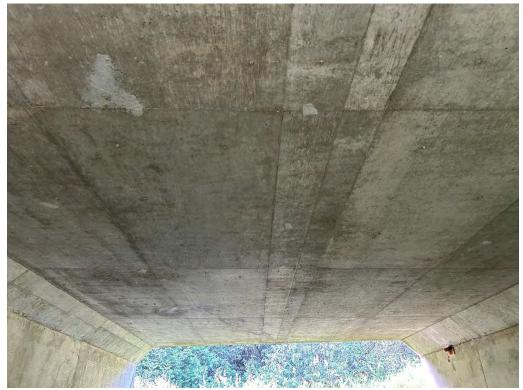
Soffit Interior - Water Staining on Ends, Light Honeycombing
