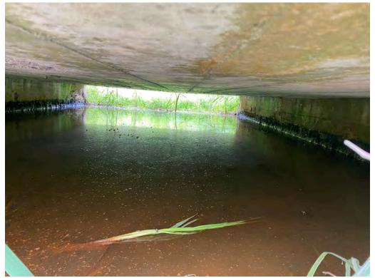
Soffit Interior - Spalls, Delaminations, Staining
