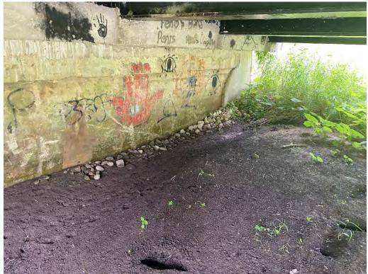
**Abutment Wall – Stained Vertical Cracks**
