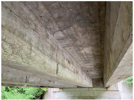
Girders – Exposed Corroded Rebar
