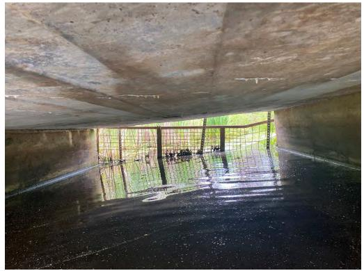
Soffit Interior - Narrow Cracking with Efflorescence, Dampness
