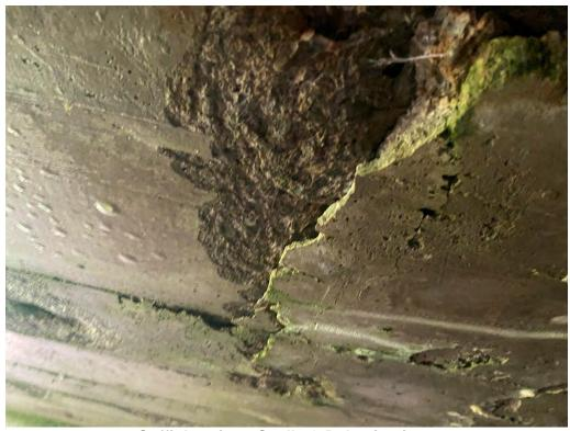
Soffit Interior - Spalls & Delaminations
