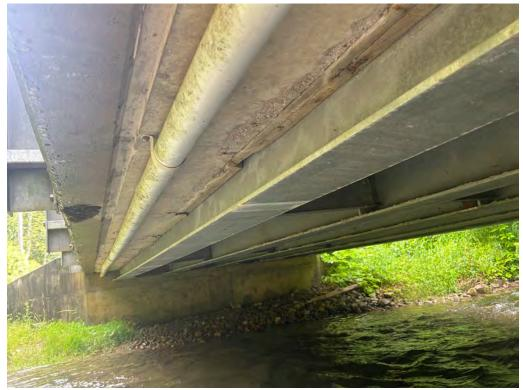
Soffit (Exterior) - Hairline Stained Cracks
