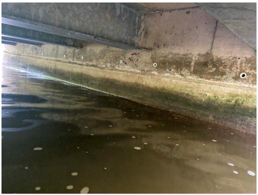
Abutments – Staining at Waterline
