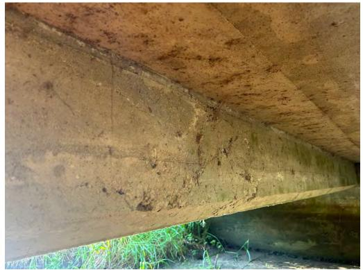
Girders Middle - Honeycombing, Hairline Cracking, Water Staining
