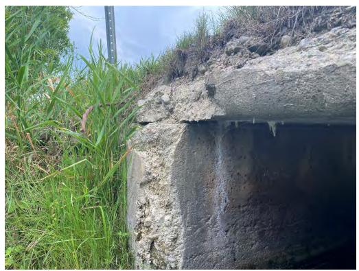
Wingwalls - Severe Spalling with Disintegration
