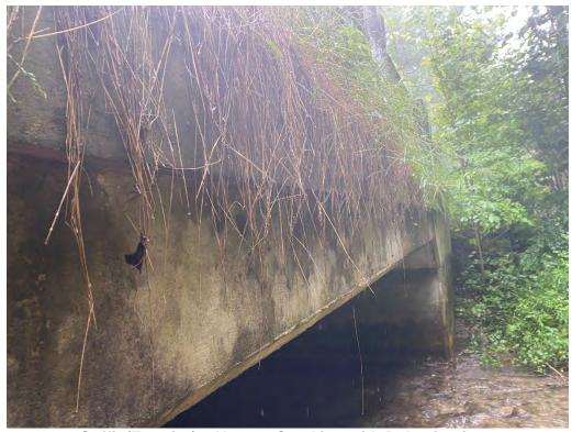
Soffit (Exterior) - Narrow Cracking with Delaminations
