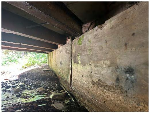
Abutments - Scaling, Water Staining, Spalling
