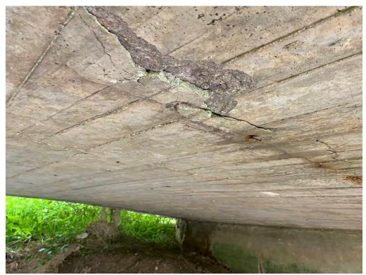
Soffit Interior – Spalling with Delaminations
