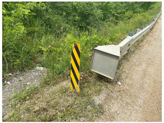
Approach Guide Rail - Impact Damage, Loose End Treatment Cables
