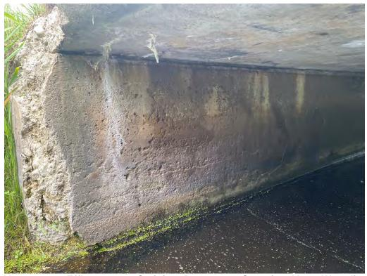
Abutments - Efflorescence Staining, Dampness, Scouring Along Waterline
