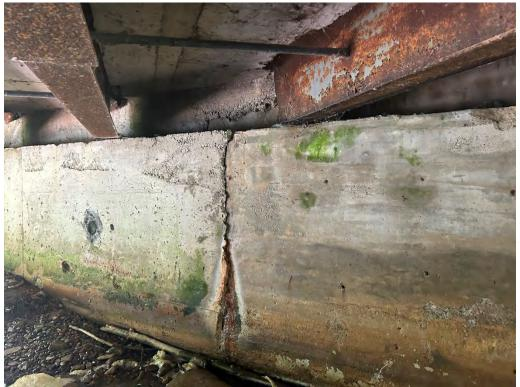
**Abutments - Cold Joints with Moisture Penetration**
