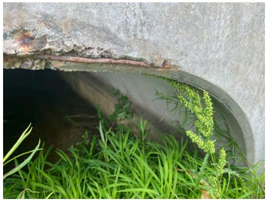
Inlet - Spalling with Exposed Corroded Rebar
