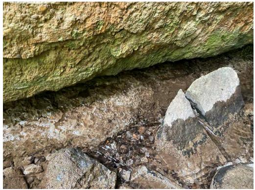
Barrel - Severe Scour at Waterline, Abutment Walls Appear to be Rotating
