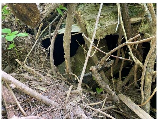
Inlet – Headwall Crushed by Trees & Debris, Severe Erosion & Undermining Behind Headwall
