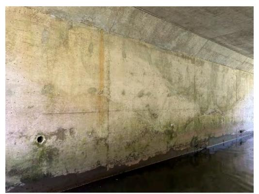
Abutment Walls - Hairline Cracking with Staining, Bug Holes, Light Scouring
