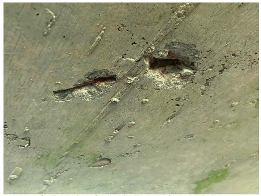
Soffit Interior – Spalls with Exposed Corroded Rebar
