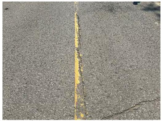
Deck Wearing Surface - Transverse & Longitudinal Cracking, Unfilled Cores
