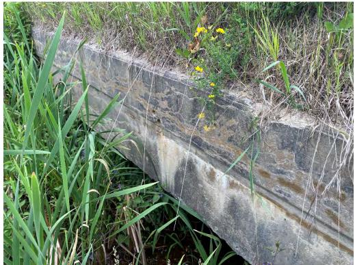
Curbs - Stained Cracking Throughout, Spalls
