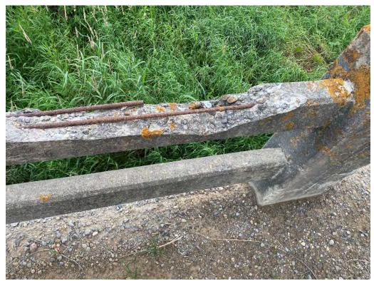
Barrier System - Spalling with Exposed Corroded Rebar
