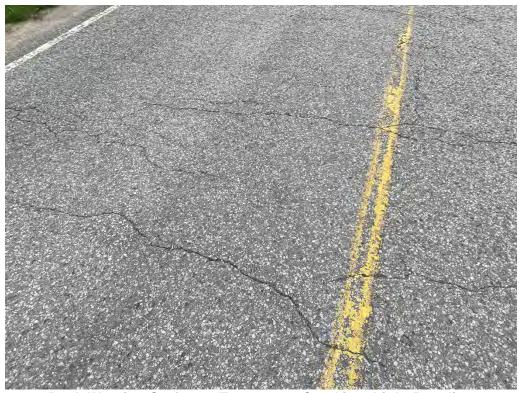
Deck Wearing Surface - Transverse Cracking, Light Raveling
