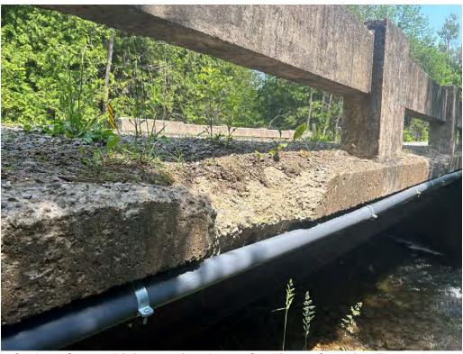
Curbs - Severe Disintegration, Large Spalling & Cracking Throughout
