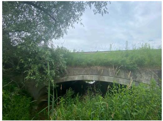
Outlet - Pattern Hairline Cracking & Staining Throughout
