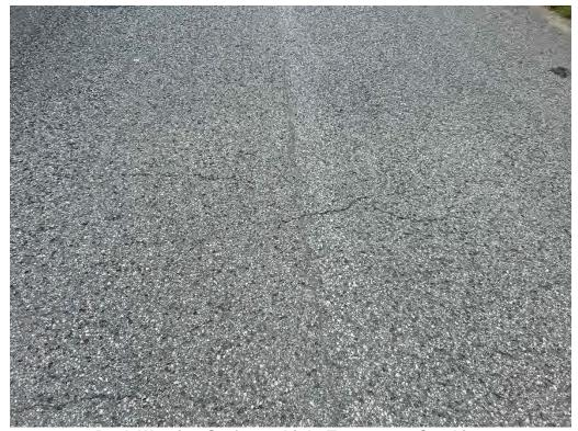
Deck Wearing Surface - Light Transverse Cracking
