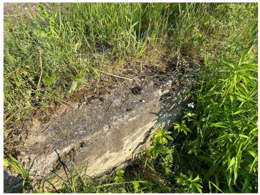
Retaining Wall - Disintegration, Delamination's, Spalling
