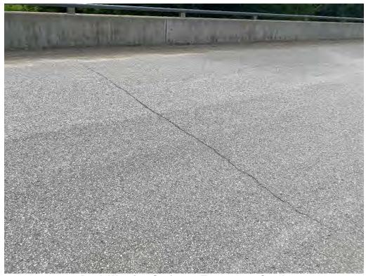
**Deck Wearing Surface – Transverse Crack**
