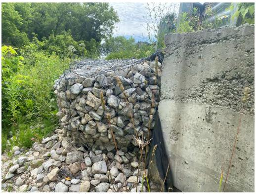
Retaining Wall – Rotation and Bulging
