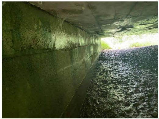
Abutments - Cold Joint with Water Staining
