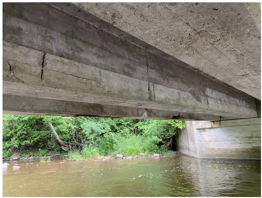
Girder – Exposed Corroded Rebar
