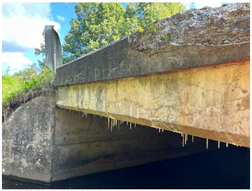
Soffit Exterior – Cracking with Efflorescence, Delaminations
