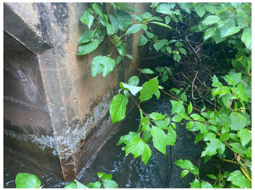
Wingwalls - Hairline Cracking Throughout, Water Staining, Scouring
