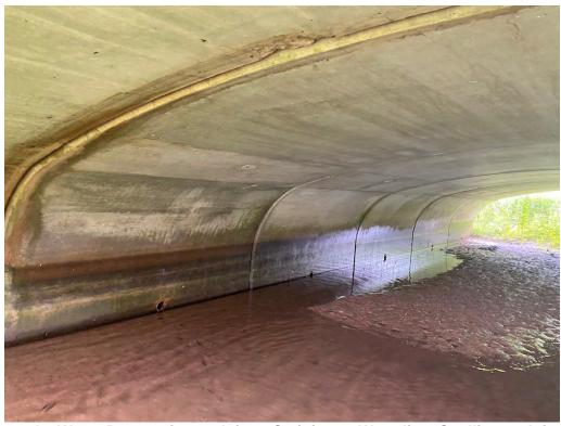
Barrel – Water Penetration at Joints, Staining at Waterline, Spalling at Joints
