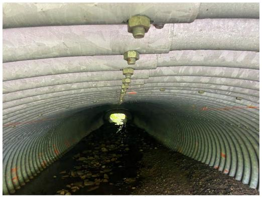
Barrel - Bulging in Panels
