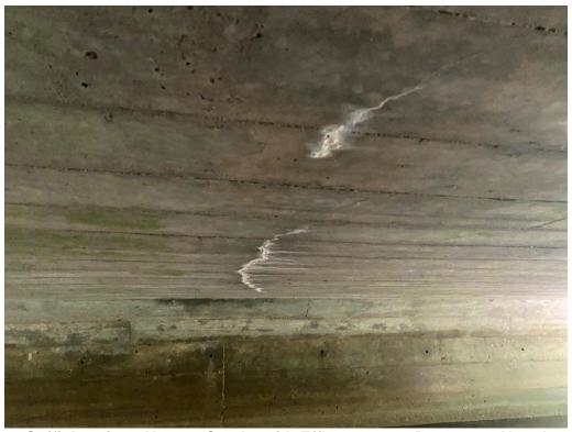
Soffit Interior - Narrow Cracks with Efflorescence, Dampness Noted
