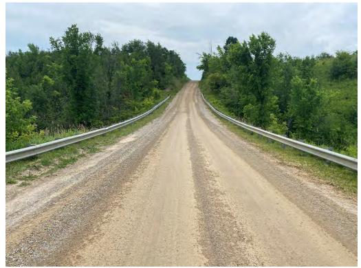
Deck Wearing Surface - Wheel Track Rutting, Loose Gravel on Shoulder
