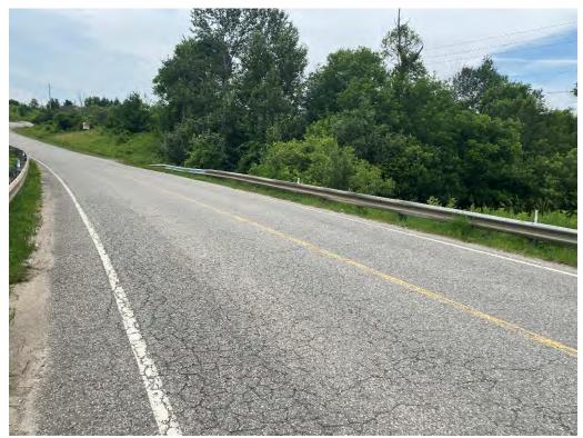
Approach Wearing Surface - Alligator Cracking, Light Abrasions
