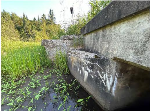
Wingwalls - Disintegration, Delamination's, Cracking with Efflorescence
