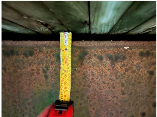
Soffit Interior - Deck Not Fastened to Girders
