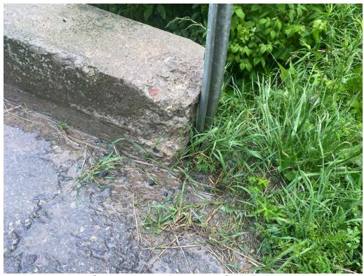
**Curbs – Impact Damage at Curb Ends**
