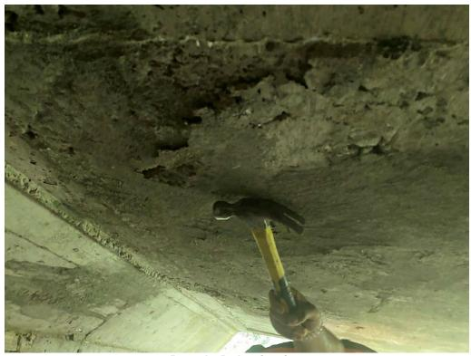
**Barrel - Delamination**
