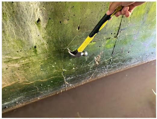
**Abutments – Hairline Stained Map Cracking & Delaminations**
