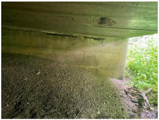
Abutments - Spalls with Exposed Corroded Rebar
