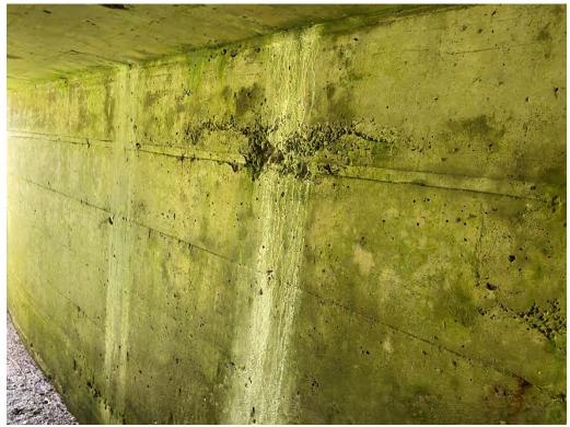
Abutments - Honeycombing, Efflorescence
