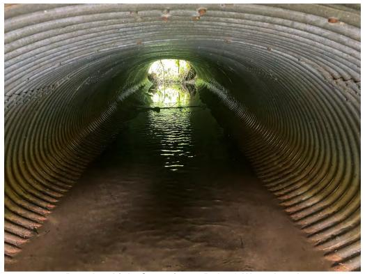
Barrels – Light Corrosion at Bolts & Water Level
