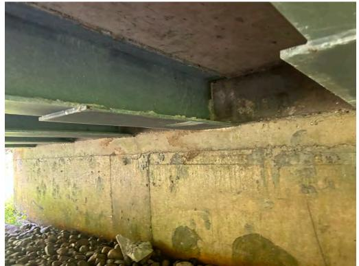
Abutment Wall - Hairline Vertical Cracks
