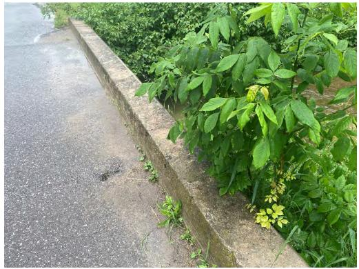
Curbs - Narrow Cracking & Staining Throughout
