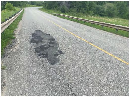
Approach Wearing Surface - Alligator & Transverse Cracking
