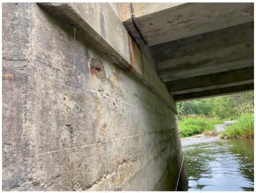
**Abutment Wall - Minor Erosion and Delaminations**
