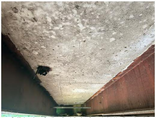
Soffit Interior – Scaling, Deck Drains Corroded & Not Functional
