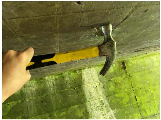
Soffit Interior - Spalls & Delamination
