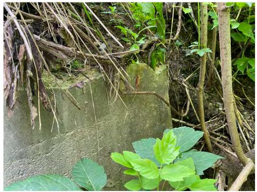
Outlet - Large Spall & Disintegration
