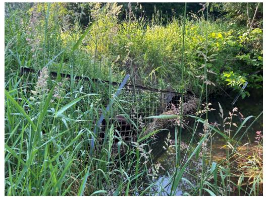
Inlet - Moderate Surface Corrosion, Several Vertical Grate Bars Cut
