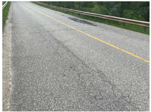
Deck Wearing Surface - Transverse & Longitudinal Cracking
