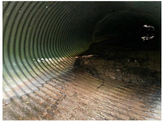
Barrels - Sag in Profile, Corrosion at Water Level, Separation at Joints
