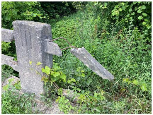
Barrier System - Severe Impact Damage
