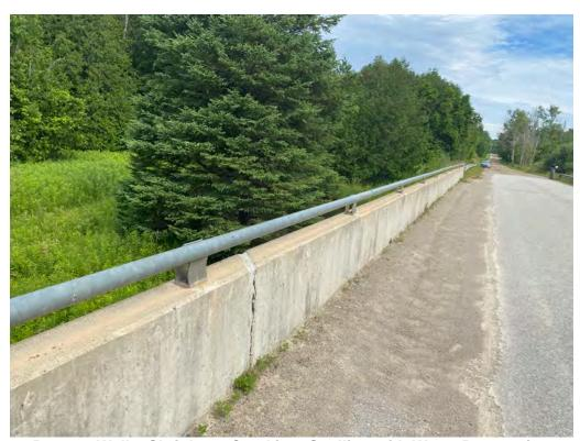
Parapet Wall – Shrinkage Cracking, Spalling with Water Penetration
