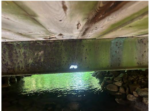
Girders Middle - Corrosion & Perforation
