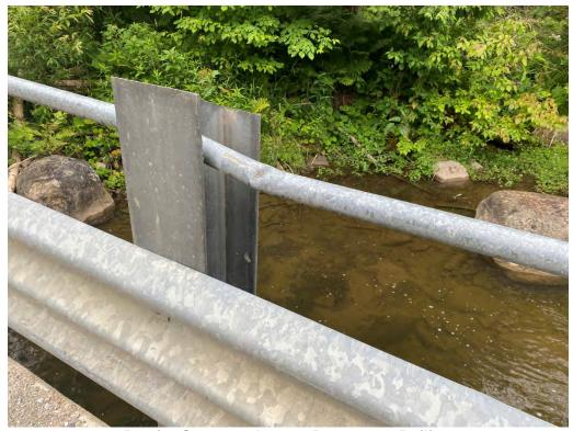
Barrier System - Impact Damage to Railing
