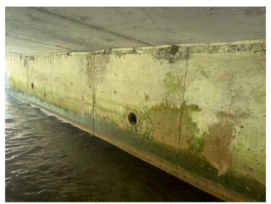
Abutment Walls - Bugholes. Spalls with Exposed Corroded Rebar, Delaminations
