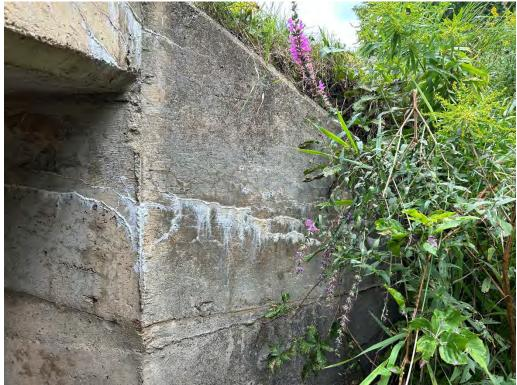
Wingwalls - Disintegration, Delaminations, Cracking with Efflorescence
