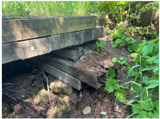
Abutments - Rotting & Deterioration
