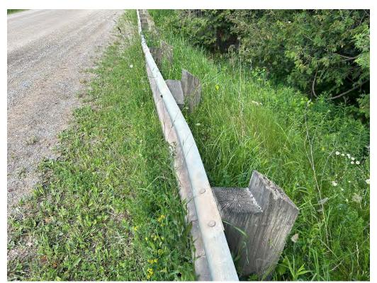
Approach Guide Rail - Impact Damage, Low Rail Height, Damaged Offset Blocks
