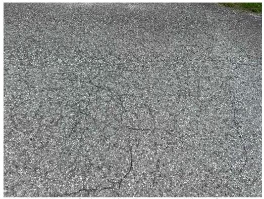
Deck Wearing Surface - Light Transverse & Alligator Cracks
