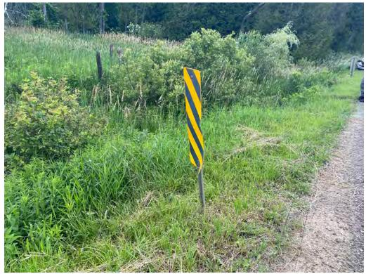
Signs – Impact Damage, Rotated, Reflectivity Weathered
