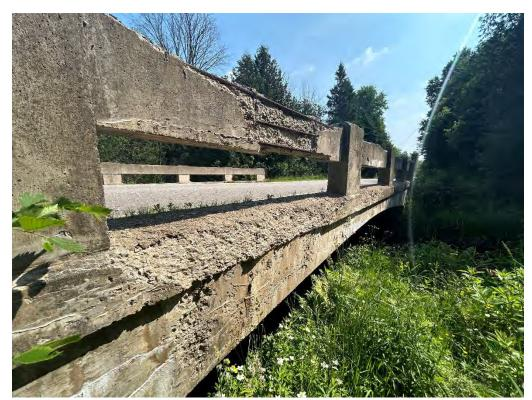
Barrier Exterior - Severe Disintegration, Exposed Corroded Rebar, Delaminations
