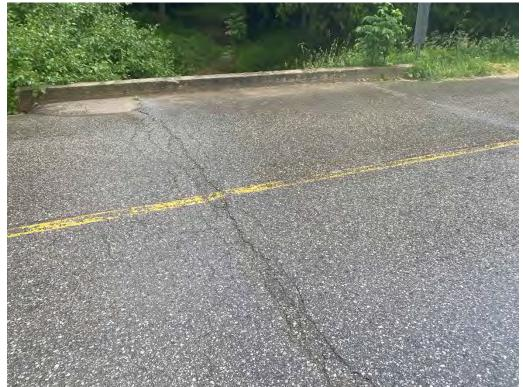
Deck Wearing Surface - Transverse Cracking, Light Ravelling, Settlement
