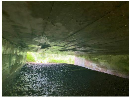
Soffit Interior – Water Staining & Honeycombing Throughout
