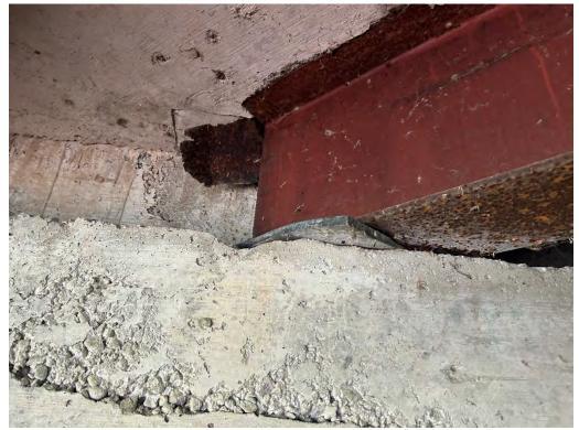
Bearings - Lack of Bearing Area, Bulging, Unevenly Loaded
