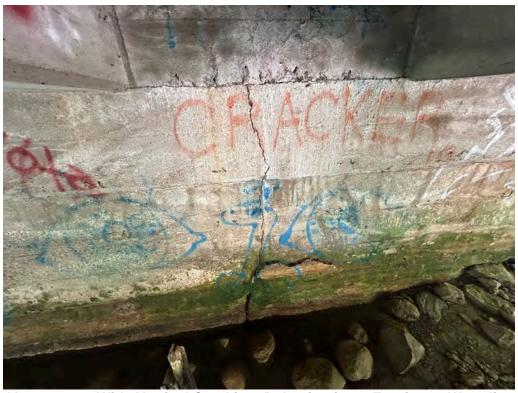
Abutments - Wide Vertical Cracking, Delaminations, Erosion at Waterline
