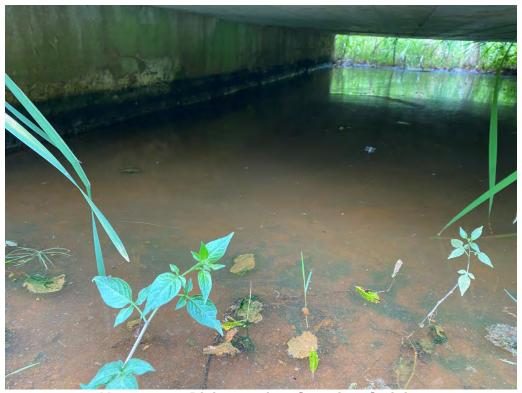
Abutments - Disintegration, Scouring, Staining
