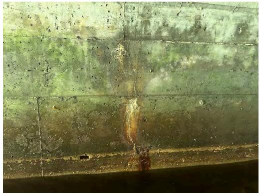
Abutment Walls – Vertical Cracking with Efflorescence
