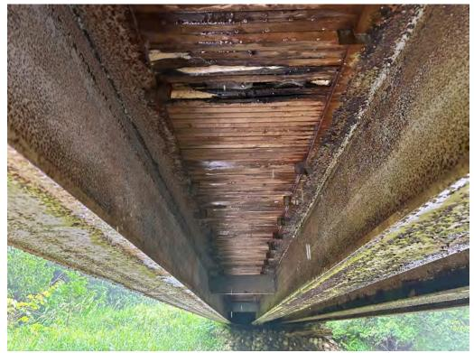
Girders - Surface Corrosion, Flaking
