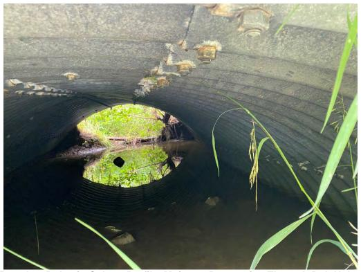
Barrels - Bulge in Culvert Profile, Moisture Penetration Through Bolt Holes
