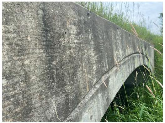
Inlet - Pattern Hairline Cracking with Staining
