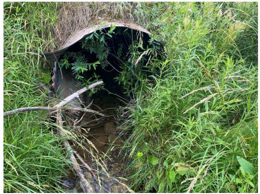
Barrels - Plate Damage/Deformation
