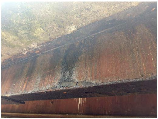
Girders Middle - Severe Rusting & Corrosion
