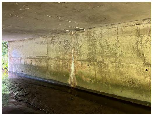
**Abutments – Wide Vertical Cracks with Efflorescence**
