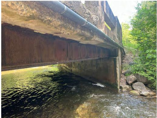
Soffit Exterior – Severe Disintegration, Delaminations & Spalling with Exposed Corroded Rebar
