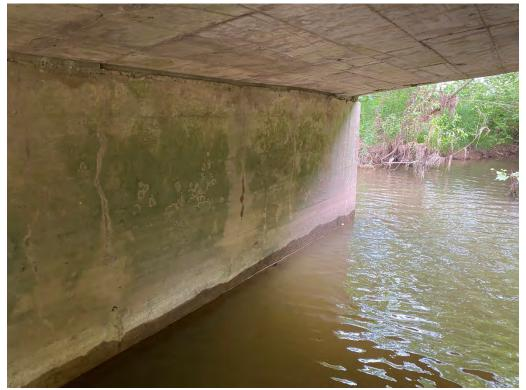
**Abutments - Stained Hairline Cracking Throughout, Dampness**
