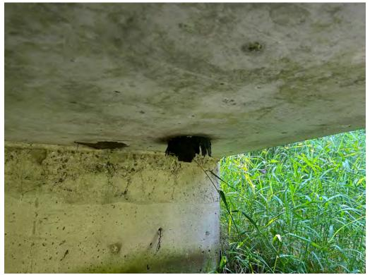
Deck Drains - Severely Corroded Downspouts, Paved Over, Not Functional
