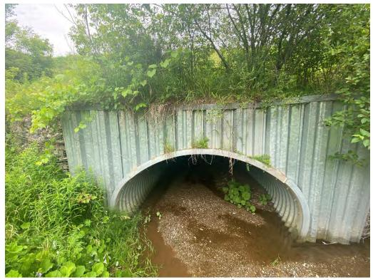
Inlet - Sheet Piling Rotating Outwards, Corrosion at Waterline
