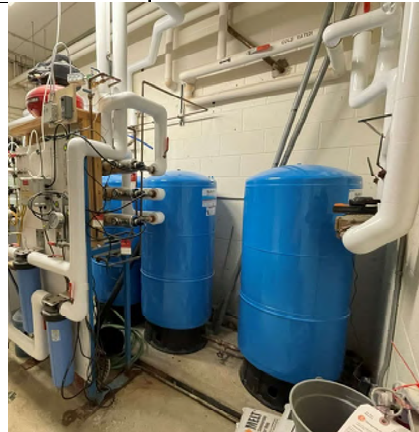
Figure 5 Three new water pressure tanks in the mechanical room
