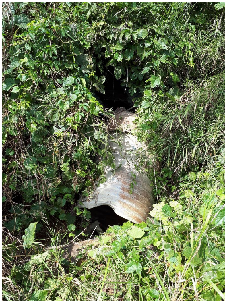
Photo 11. One of a series of dilapidated culverts.
